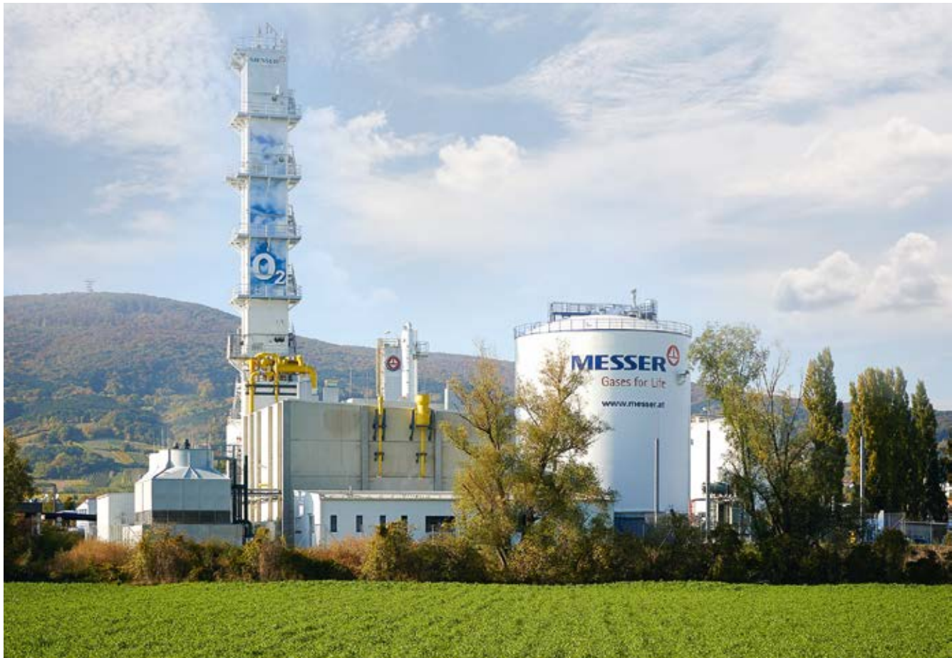
Air separation units exclusively process ambient air for use in the production of industrial gases.
